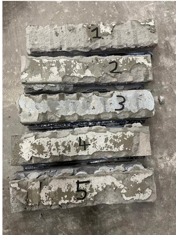
Plate 12 - Bond Strength Failed Brick from HURST TRACKWALL Brick Slip Cladding System
