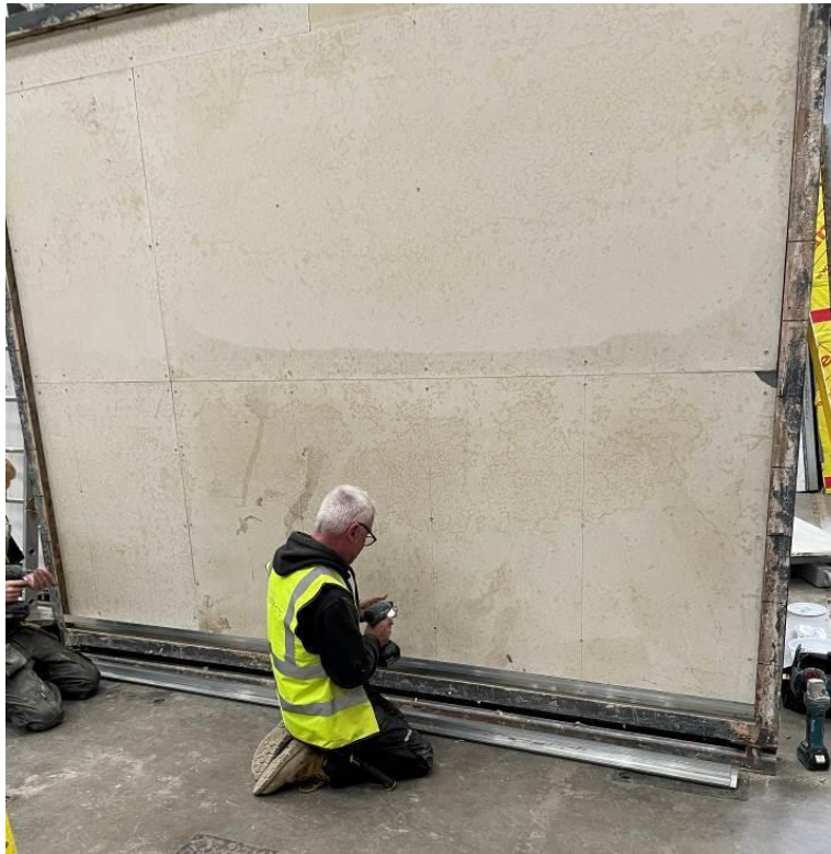
Plate 3 – Application of 'Z' Rails Upon Y-Wall
