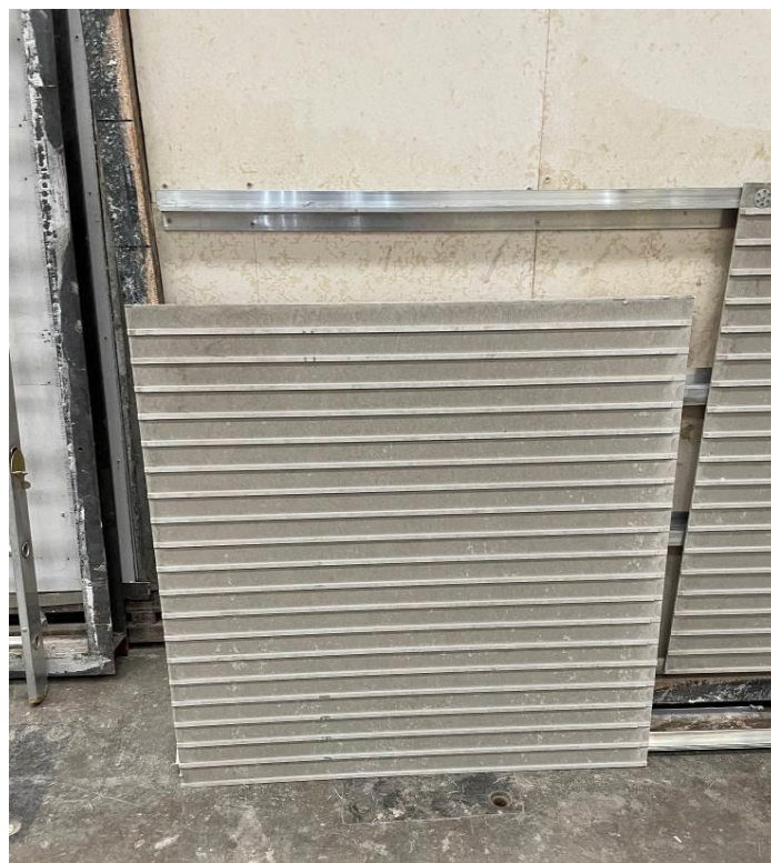
Plate 4 – Fixing of Brick Slip Carry Board Upon 'Z' Rails
