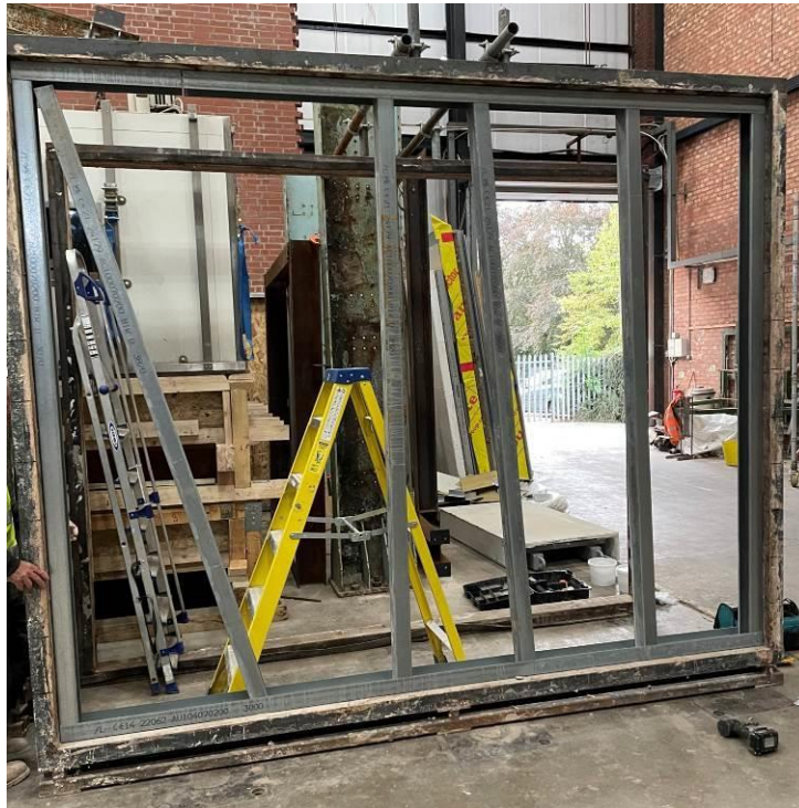
Plate 1 – Installation of Base and Support Rails
