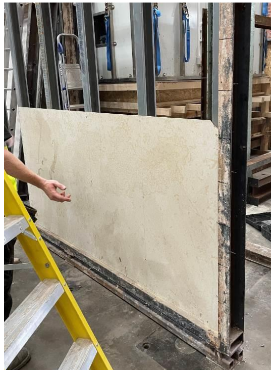
Plate 2 – Application of Y-Wall Boards to Base and Support Rails
