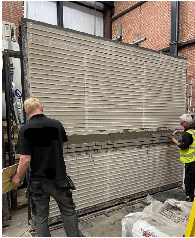
Plate 5 – Application of Tile Adhesive and Brick Slips
