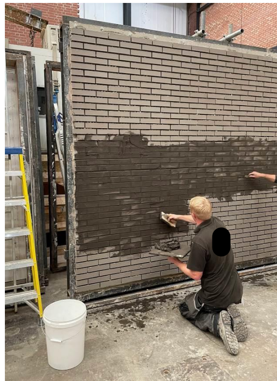
Plate 6 – Application of Plasticizer and Cement Mixture
