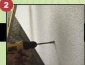
Drill a 16-18 rom hole through the render and insulation until the original substrate is reached.
