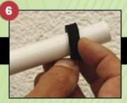
Insert SWI-ST place washer and Drill through tube into substrate to the appropriate depth for fixing (site specific).
