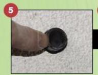
Insert extension tube into system back to substrate.
