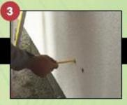
Insert tube, or measure depth of hole from finished render back to the original substrate, making an allowance of dram to allow the neoprene washer to compress and provide a seal when installed.
